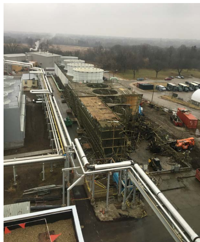
Cooling tower demolition
