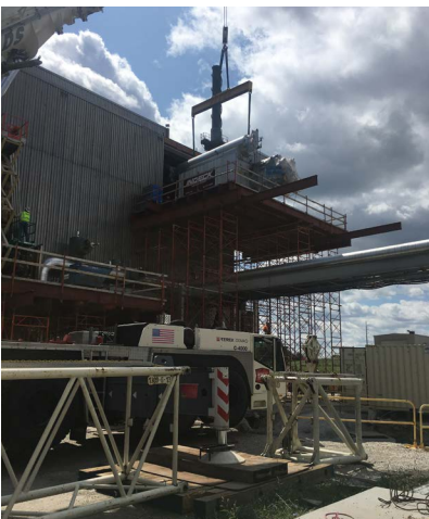
New boiler installation
